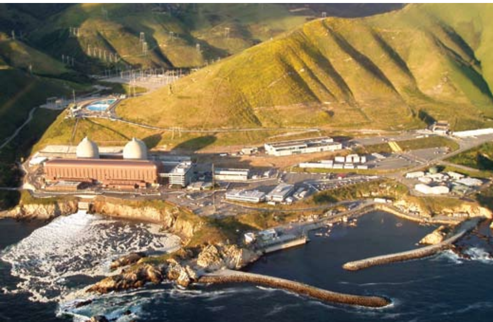
Diablo Canyon Nuclear Power Plant. Photo: emdot_marya
